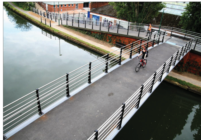
Not only did the new "Grand Union Bridge" facilitate significant improvements for pedestrian and cyclist access to the Grand Union Canal, near Alperton, it was unique in its overarching objectives and aspirations to design out crime.
