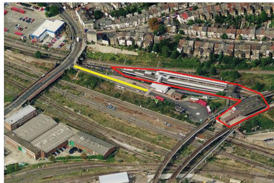
Willesden Junction – a recognised ‘interchange’ station set in a poor urban realm. Large swathes of railway track and associated land take lead to accessibility and general environmental issue. The (split-level) station is outlined in red, the key access point ‘Station Approach’ is lined in yellow. It is critical that a new international High Speed Railway station at Old Oak Common (to the south) links by way of a travelator, similar to those operating in airports, illustrated here:
